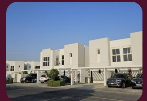
Project Name: Mudon Arabella 03 - 509 Villas Location: Damac Hill Client/Owner: Dubai Properties / North 25ICD / Ithra Consultant: Lacasa Contractor: Beaver Gulf Contracting
