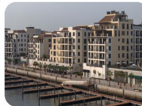
Project Name: Port De La Mer Phase 2 (4 Buildings G+6), Plot 03 Location: La Mer, Jumeira Client/Owner: Meraas Consultant: Dewan Contractor: Beaver Gulf Contracting
