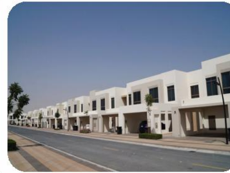
Project Name: Nshama 2452 Nos of Townhouses (Zahra, Hayat, Noor, Naseem & Sama) Location: Al Qudra Client/Owner: Nshama Consultant: Arif & Bint oak Contractor: Beaver Gulf Contracting
