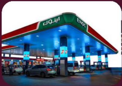
Project Name: ENOC Filling Stations – 1021,1064 & 1094 Location : Al Warsan, Wadi Al Safa and Al Barsha Client/Owner: ENOC, Consultant : CHSS & BHNS Consultant. Contractor : BEAVER Gulf Contracting
